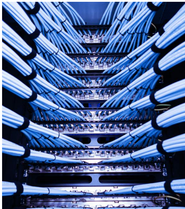
Handbook on Operational Technology and its Security Introducing an OT/OT Security Framework
